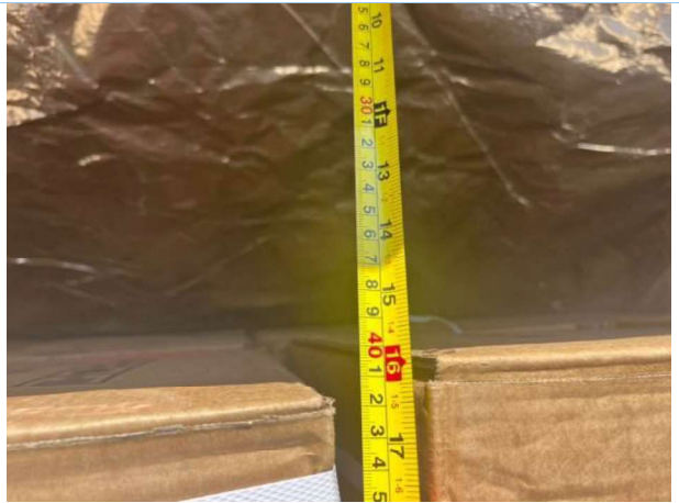
View of void space measurement at roof panel
