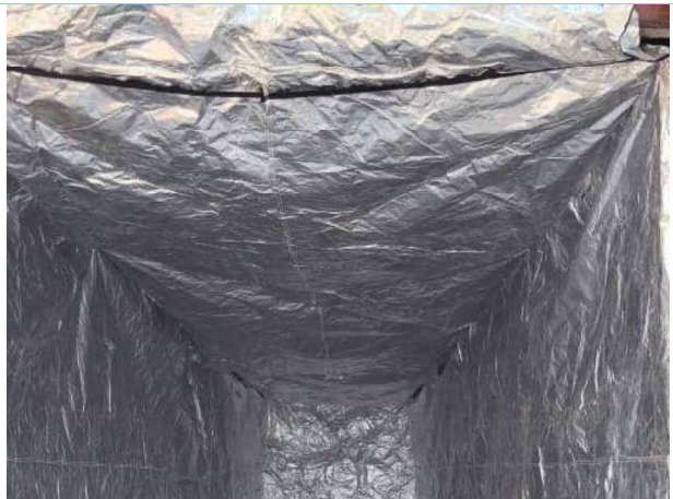
View of interior panels
