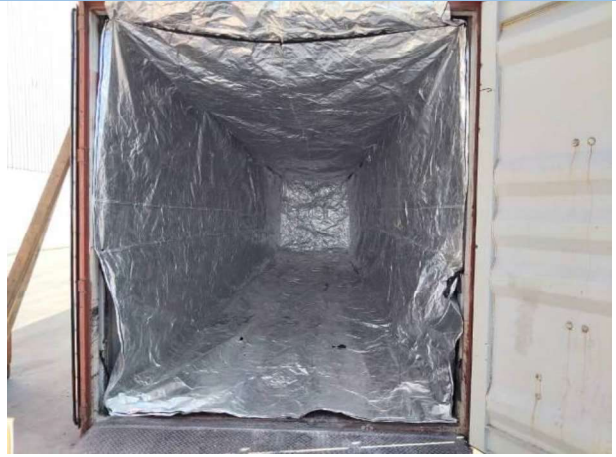
View of interior panels
